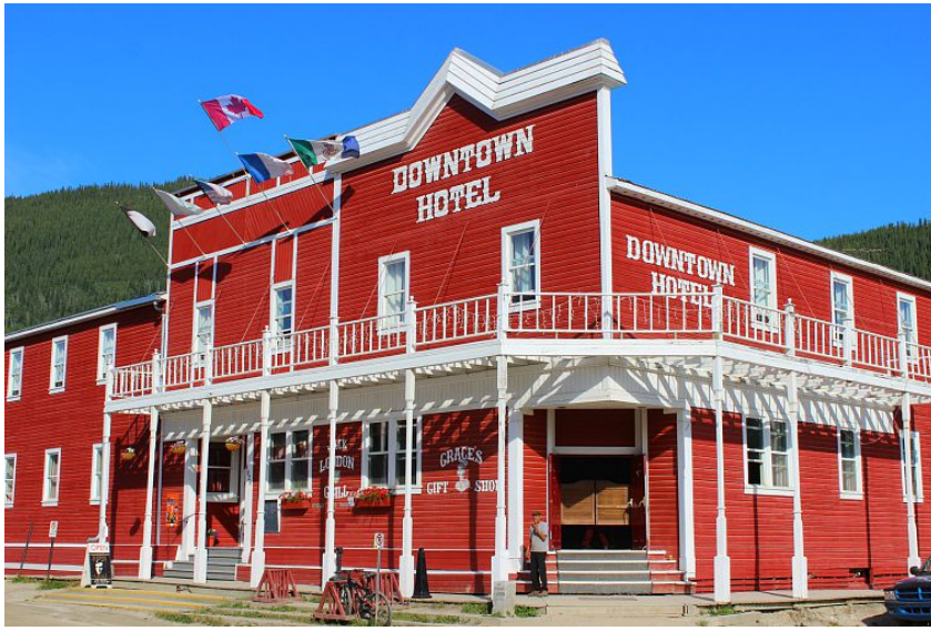
Figure 3. Downtown Hotel. Example of existing balcony over boardwalk.
