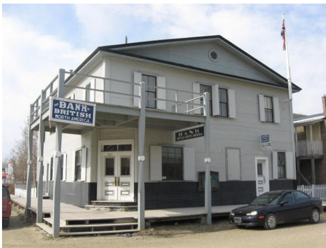
Figure 4. BNA Bank. Example of an existing balcony over boardwalk.
