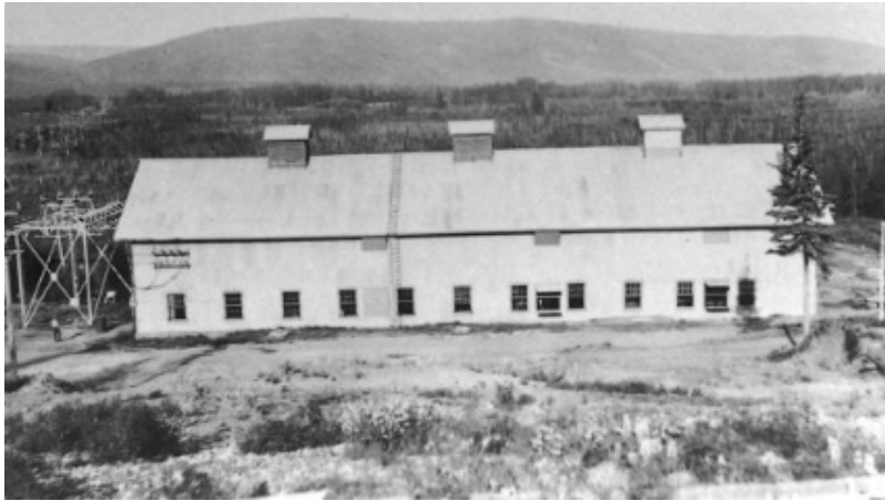
The new hydro plant 1911
