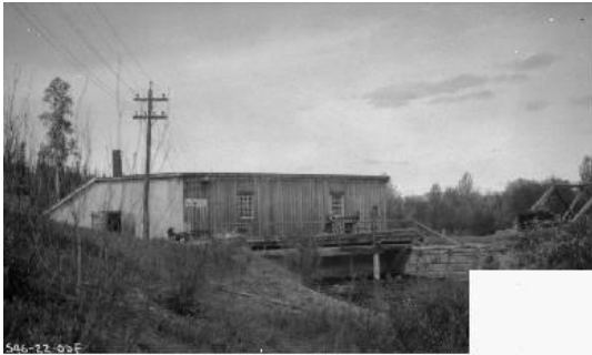
NORTH FORK INTAKE
