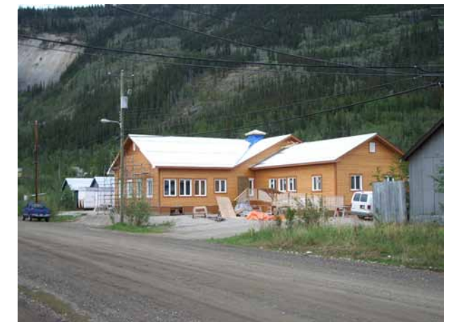
A day care centre built by the Tr'ondëk Hwëch'in on Second Avenue is one of a number of new buildings in the North End. (Photo: H. Kalman)
