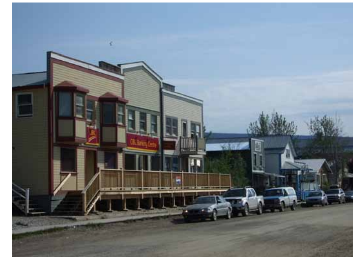
The CIBC on Second Avenue is a recent building with Gold Rush features. Its high ground floor and entrance walkway respect the flood plain but alter the streetscape. (Photo: H. Kalman)
